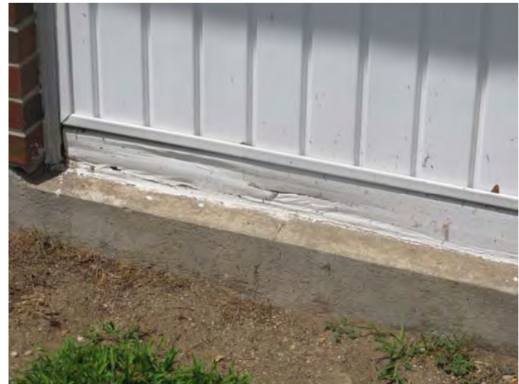
Moisture damage/deterioration widespread at window infill panels of Rosewood I buildings
