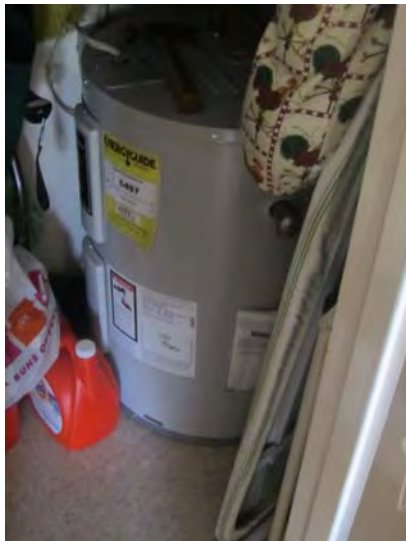
Each unit has an electric-type tank for generation of domestic hot water
