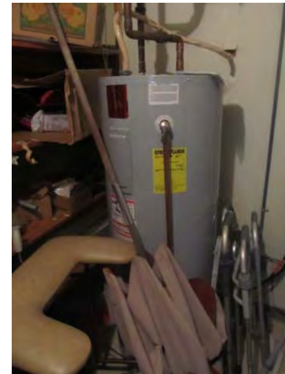
Electric domestic hot water tank serving community building – No problems observed or reported
