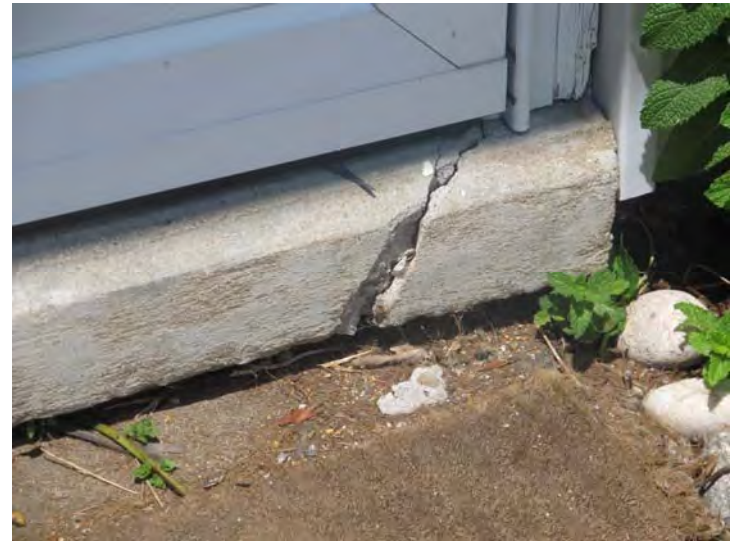
Isolated masonry surfaces in need of repair/re-pointing
