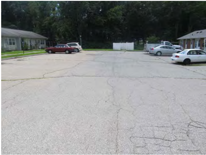
Asphalt paving at parking areas exhibits age-related cracks and wear
