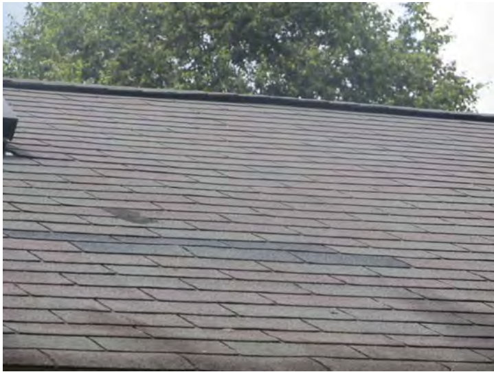
Conventional three-tab shingles on roof surfaces exhibit age-related wear
