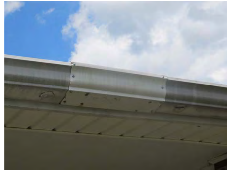
Past repair efforts noted on gutters for roof drainage systems at various locations
