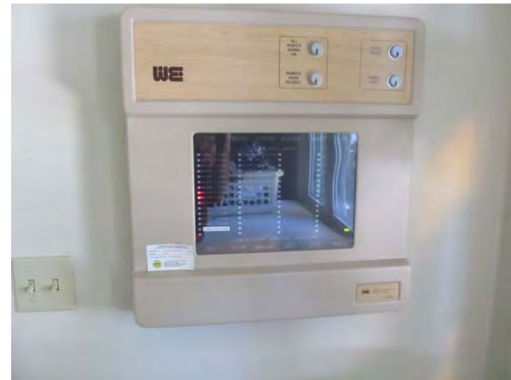
Zone-based annunciator panel for fire alarm system located at community building – Operational problems reported by management
