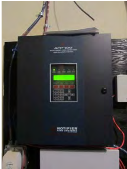
Typical building-based fire alarm panel – Management reports widespread operational problems
